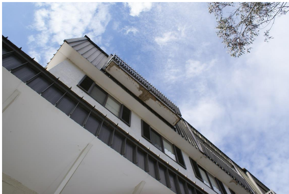
Figure 6: Photo of the existing balcony to be demolished and replaced with a deck
